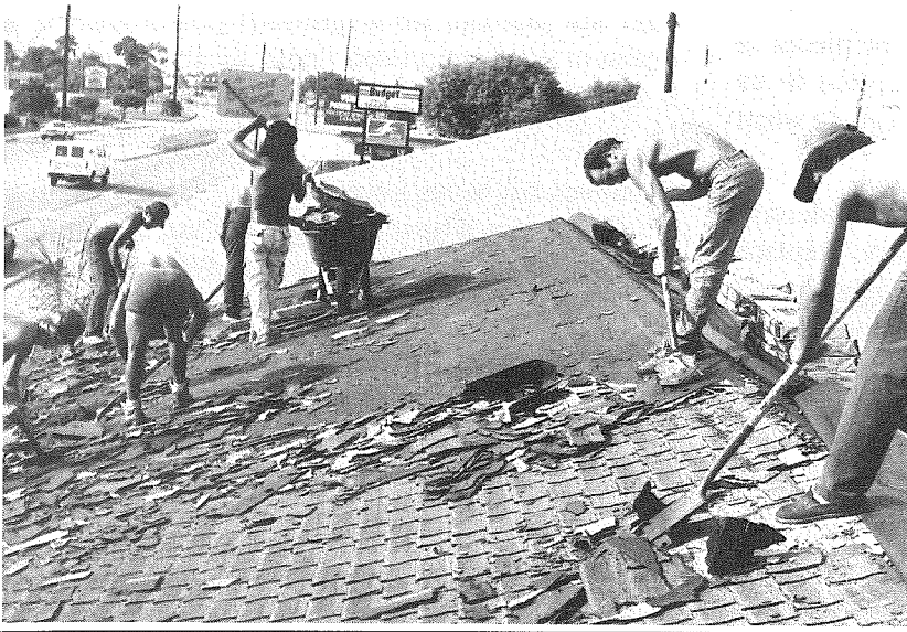
Figure 13-6 Remove shingles starting at the ridge
